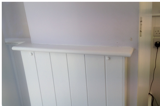
Figure 13: Easily removable wall panelling so that they do not have to be forcibly detached.
