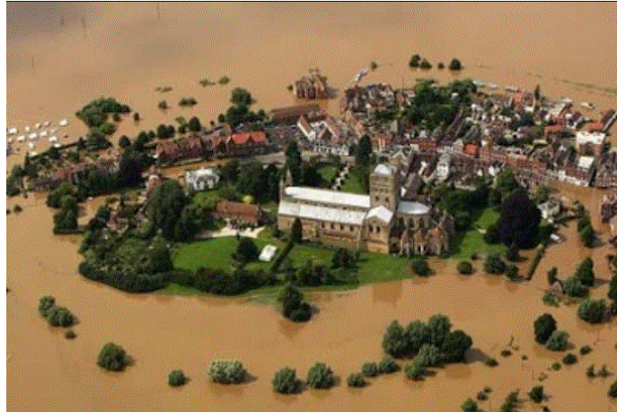
Figure 1. Tewkesbury Abbey flooding - July 2007 (BBC, 2008)
